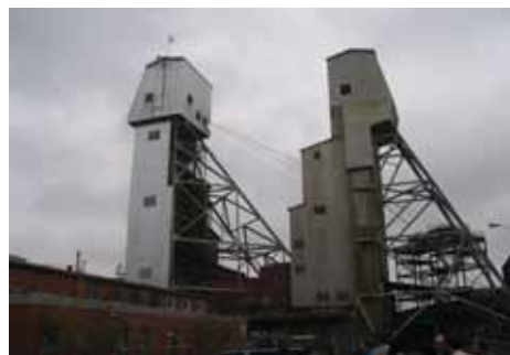
Number 7 hoisting headframe at INCO operation
